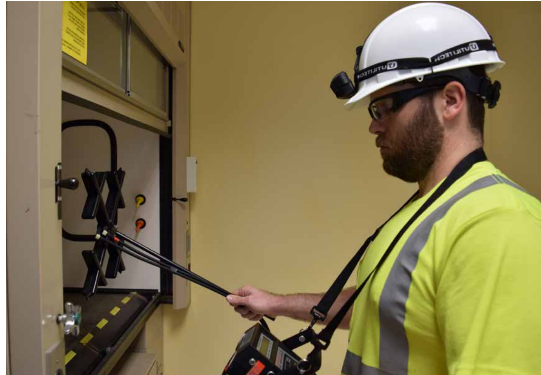
Testing fume hoods in Clark Hall to optimize the building's energy profile
