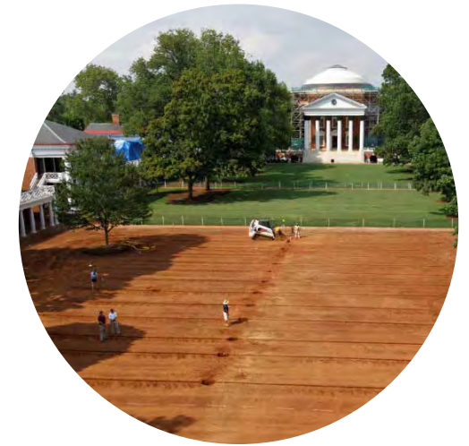
2012 sod replacement and drainage installation
