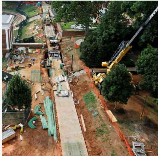
UTILITY DUCT BANK INSTALL
