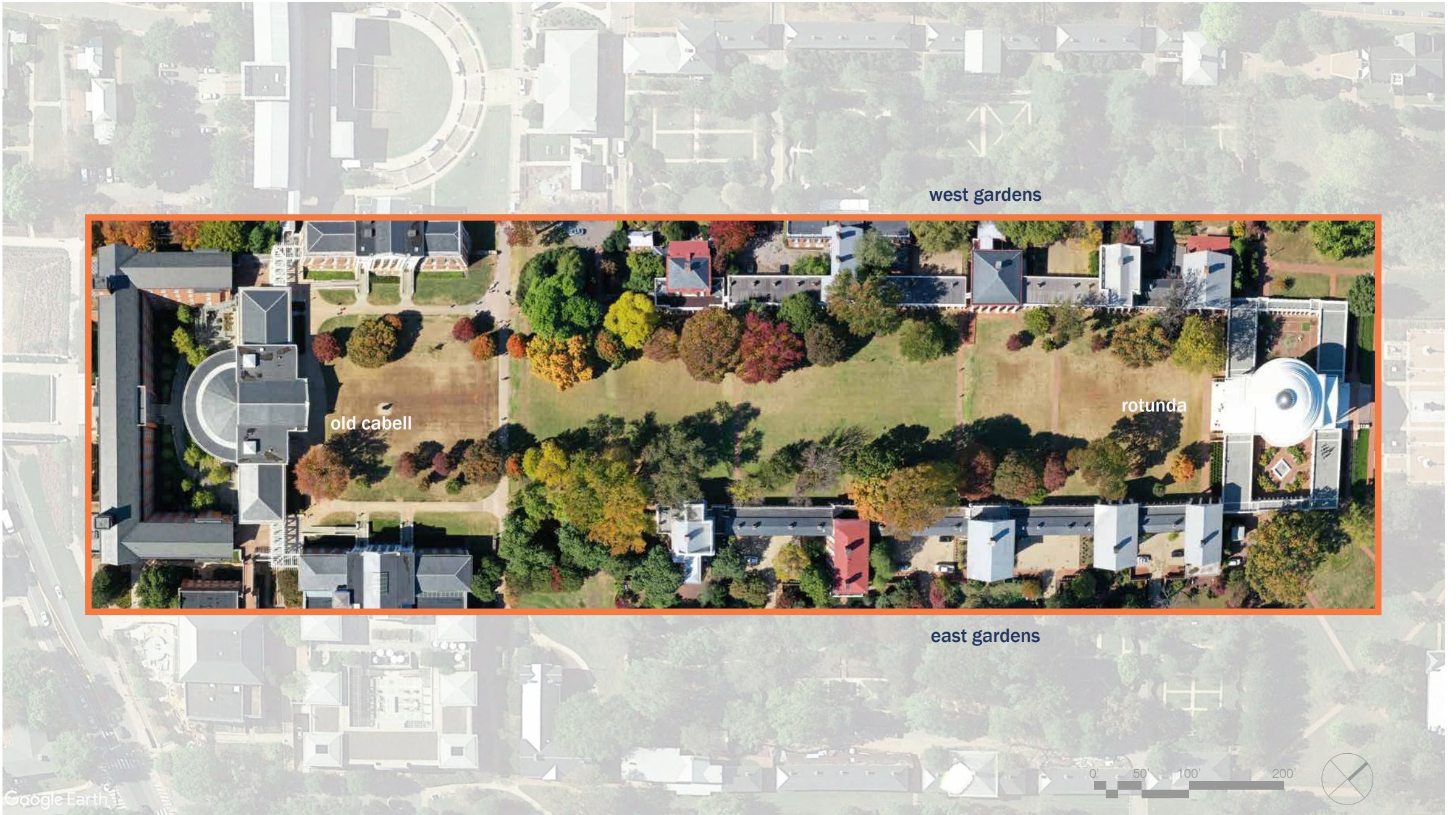
EXTENTS OF STUDY AREA | The 4.5 acre Lawn study area was flown with a drone. The aerial was captured in late October 2019.
